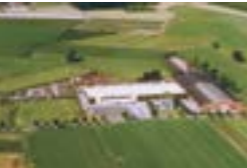
Expanding the production facility in Achtmaal
