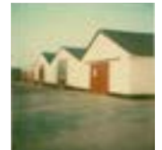
Building of a new production facility in Achtmaal
